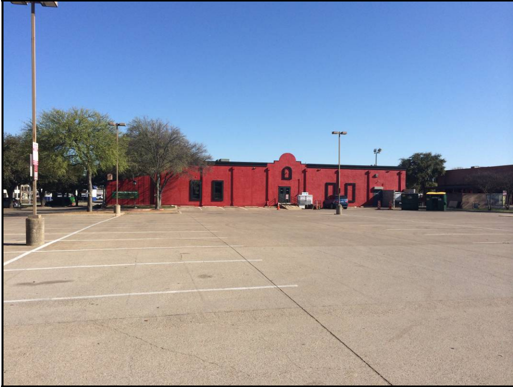
Looking northerly at subject rear.
