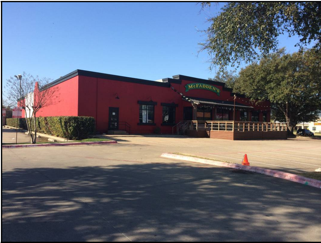
Looking southwesterly at subject.
