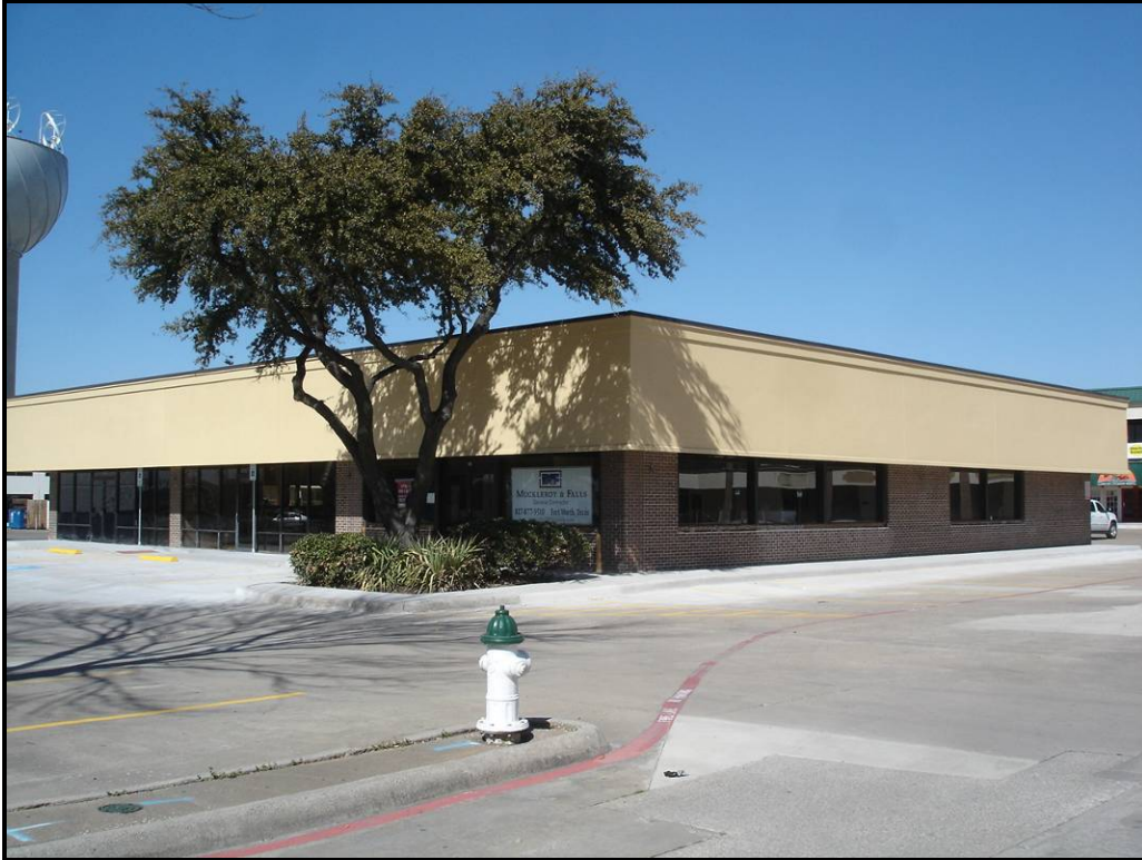
Looking northwesterly at subject improvements (retail strip center).
