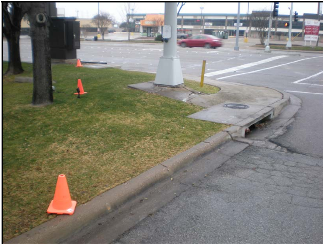
Looking northwest along the proposed fee simple acquisition.
