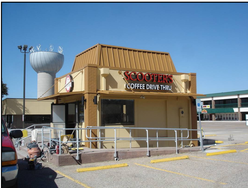
Looking northwesterly at subject improvements (kiosk building).
