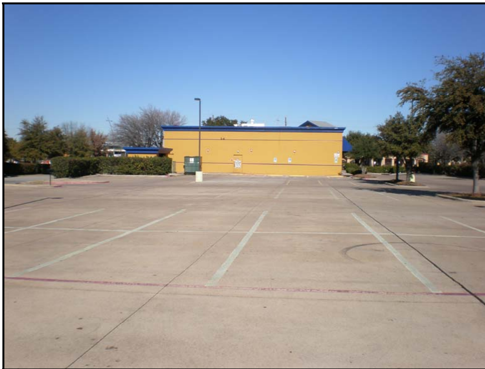
Looking north at the rear of the improvements.
