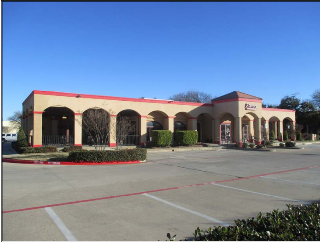
Summary view of building improvements.
