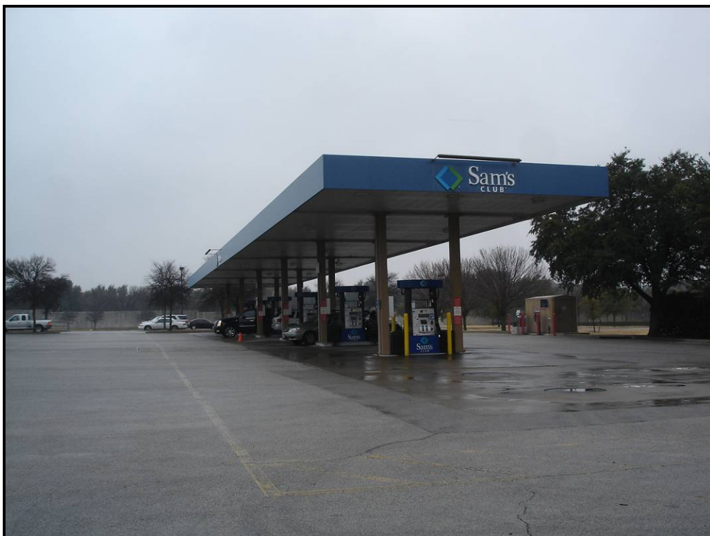
Looking southerly at subject improvements near proposed acquisition; approximately 120 feet south of acquisition area.
