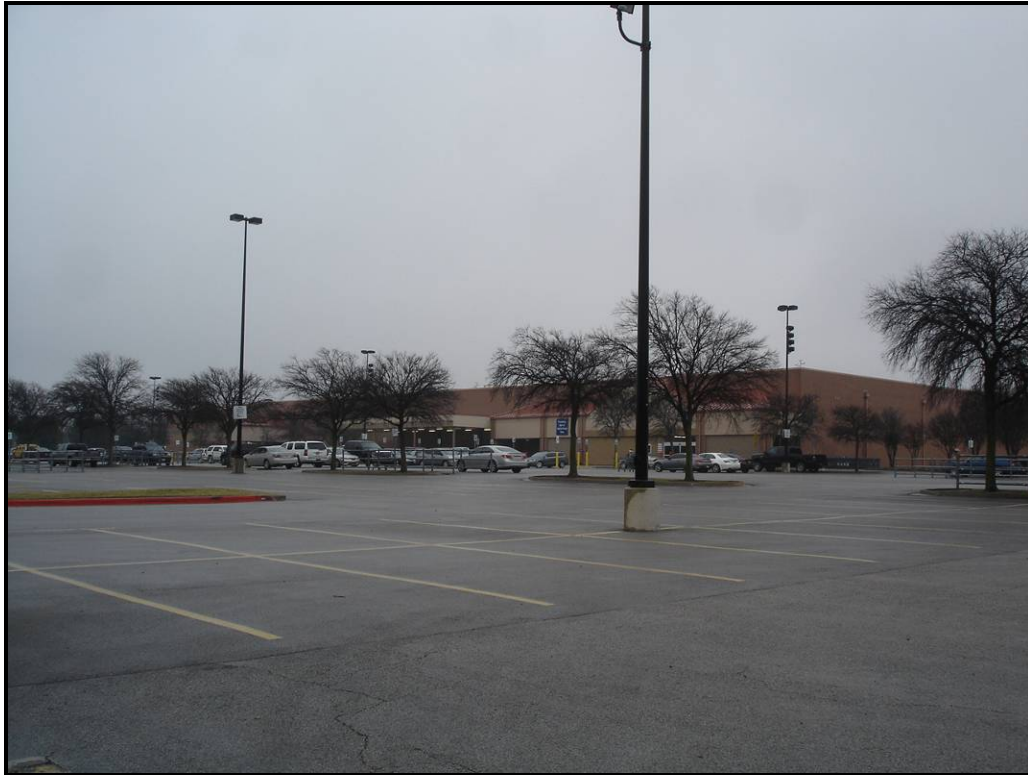
Looking southeasterly at subject improvements.
