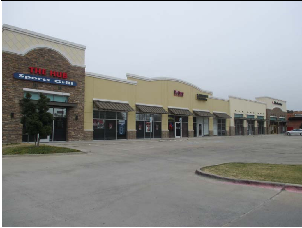
Viewing northeasterly and eastern retail building.
