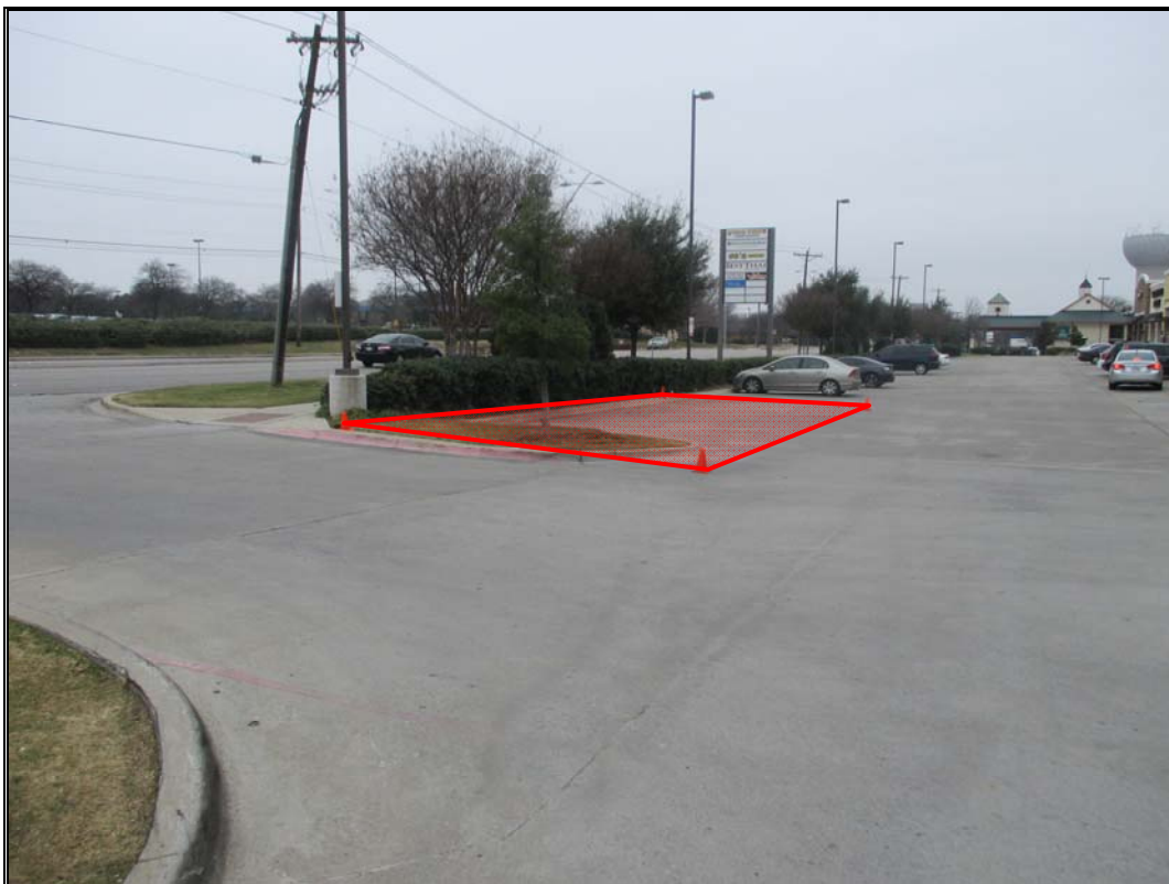
Southwesterly view of proposed acquisition encumbering parking area.
