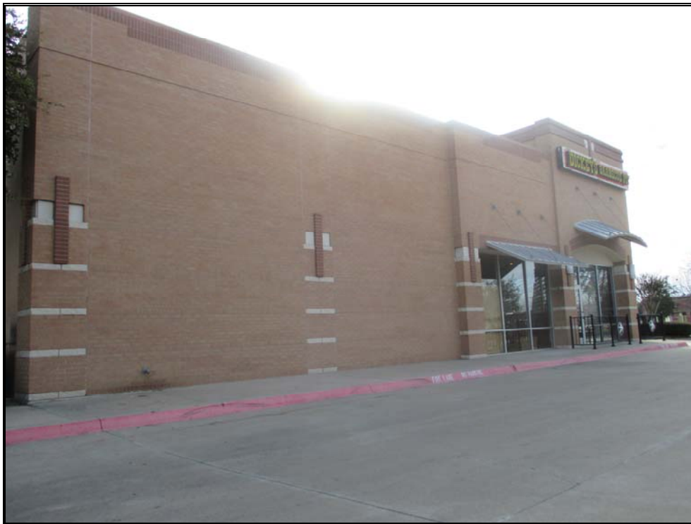
View of western side of western building.
