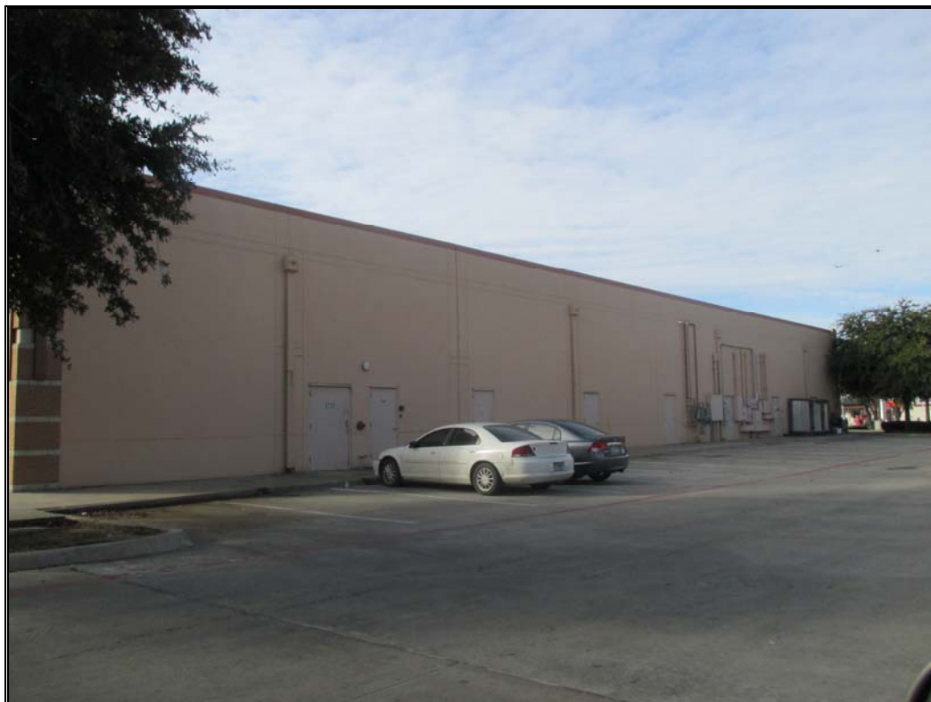
Southwesterly view of rear of eastern building.
