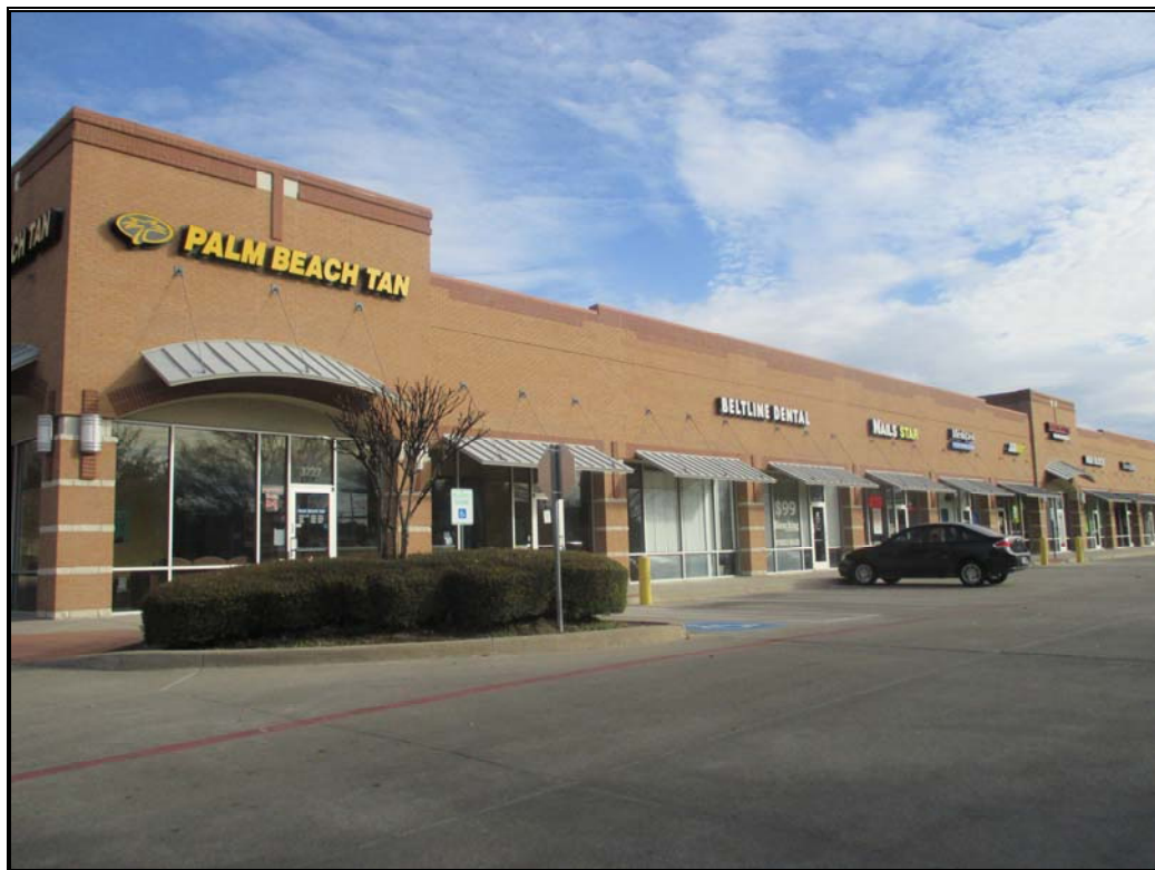
Northerly view of eastern building.
