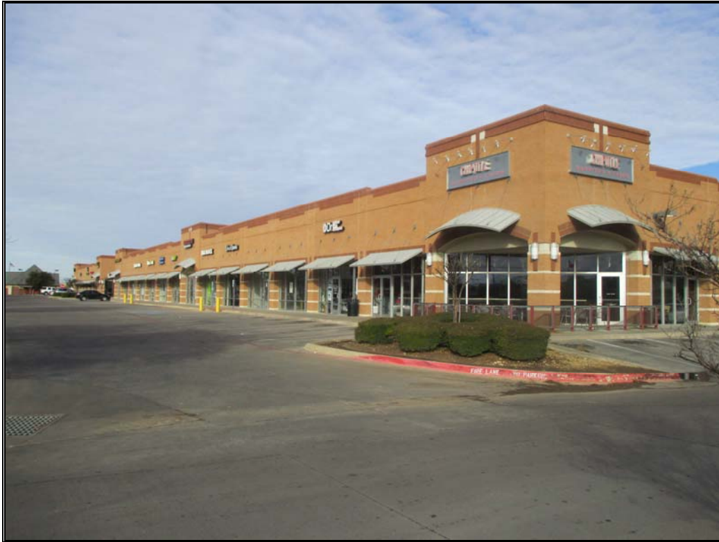
Viewing westerly, summary view of eastern building.
