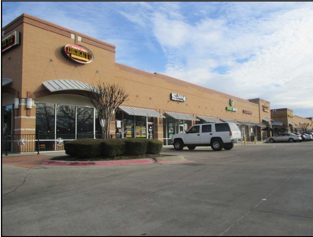
Northeasterly view of western building.
