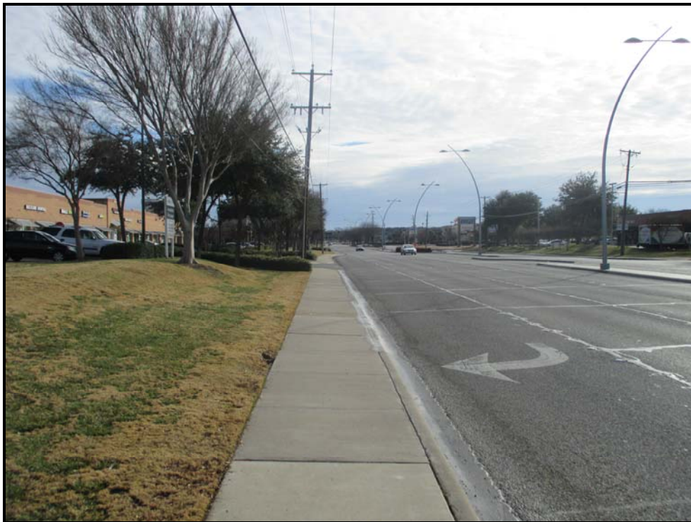
Looking easterly along Belt Line Road, subject on left.
