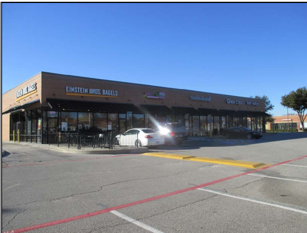
Summary view of main building improvements.
