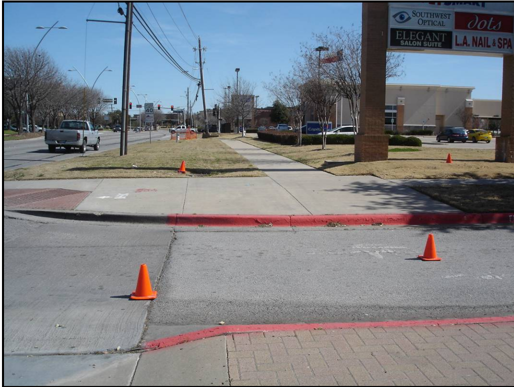
Looking easterly along existing ROW line for Belt Line Road, subject on right.
