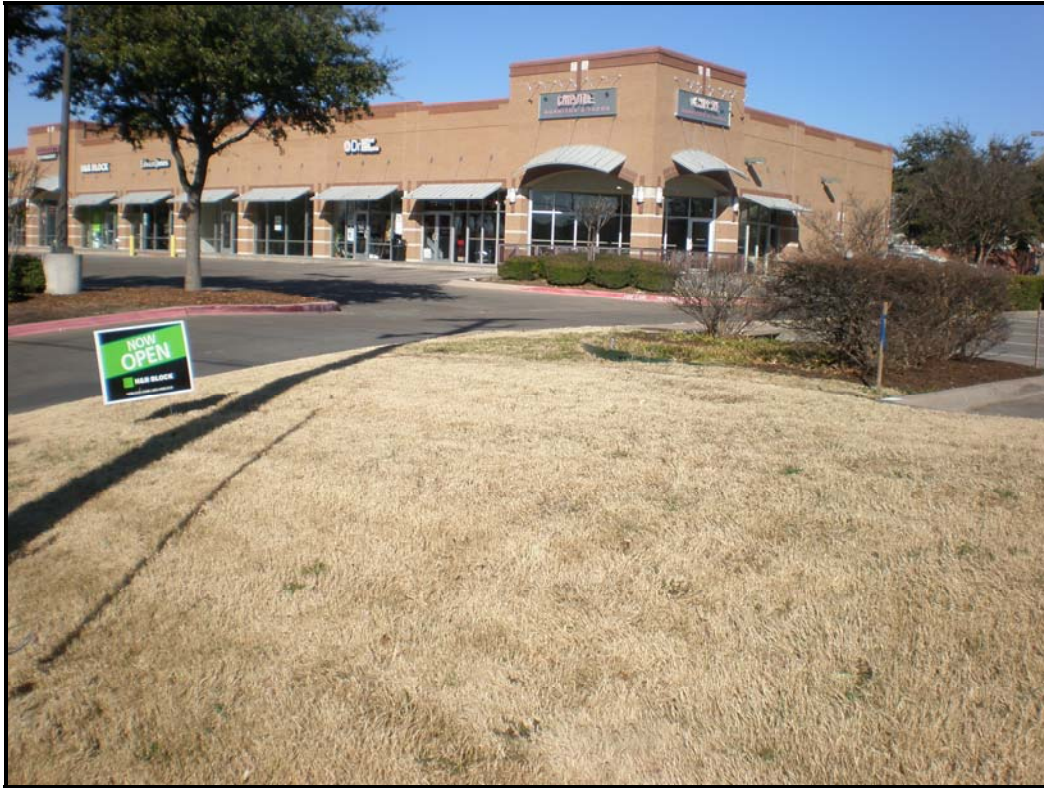
Looking northwest across the proposed permanent easement.
