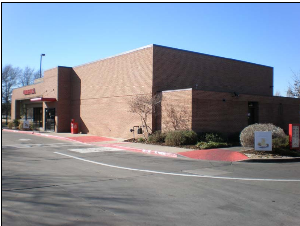
Looking south at the rear of the improvements.
