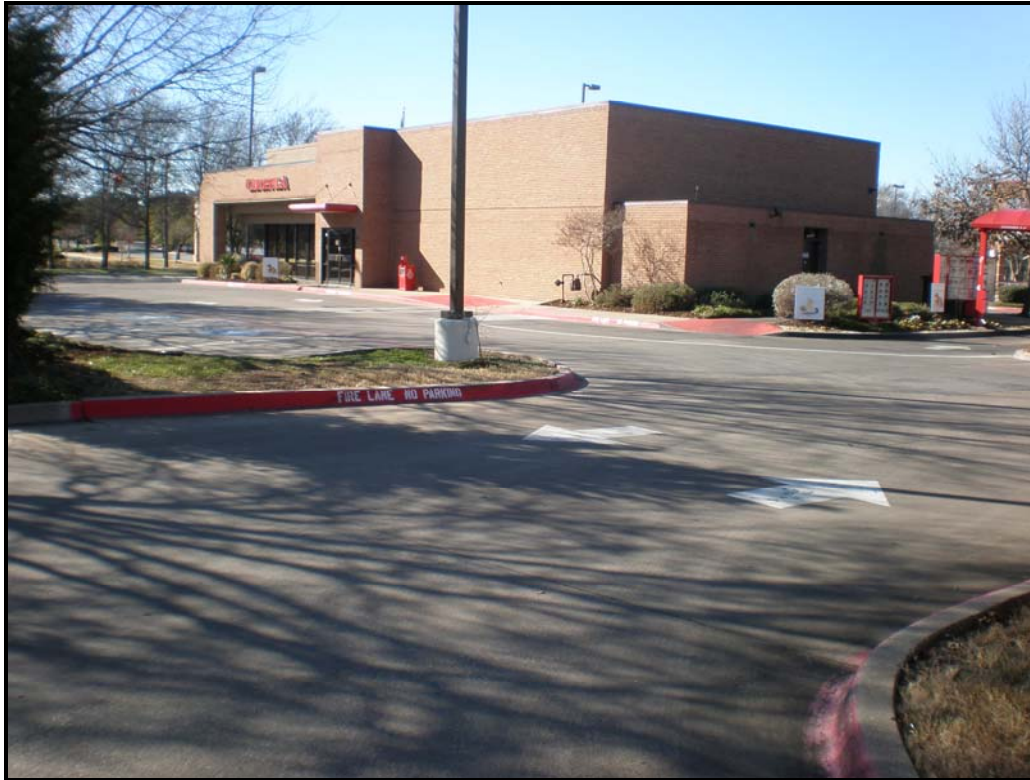
Looking southwest along the cross access with the eastern abutting property.
