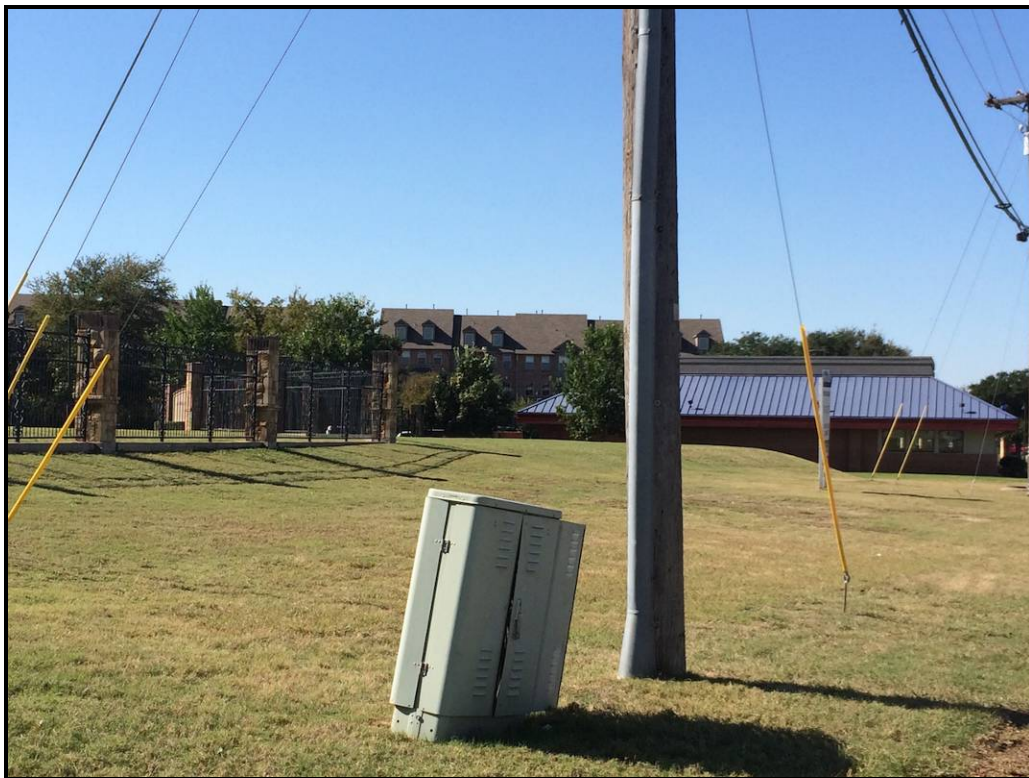
Looking southwesterly at subject property.
