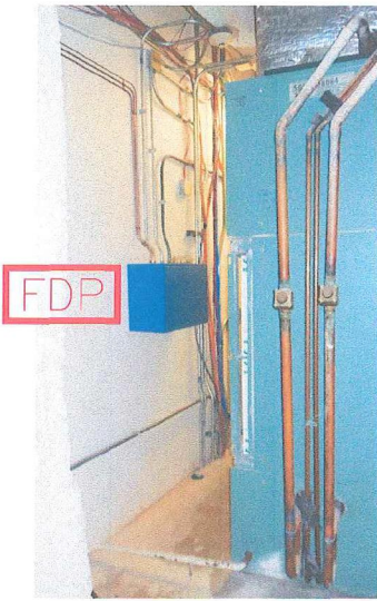
TERMINAL AND WALL MOUNT RACK INSTALLTION
