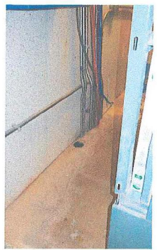
3RD FLOOR EXISTING DUCT WHERE IT WILL EXIT OUT.
