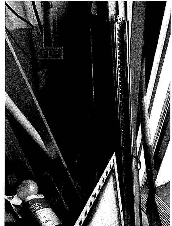
LOCATION OF NEW FPD - CUSTOMER IS TO CLEAN LOCATION PRIOR TO CONSTRUCTION
