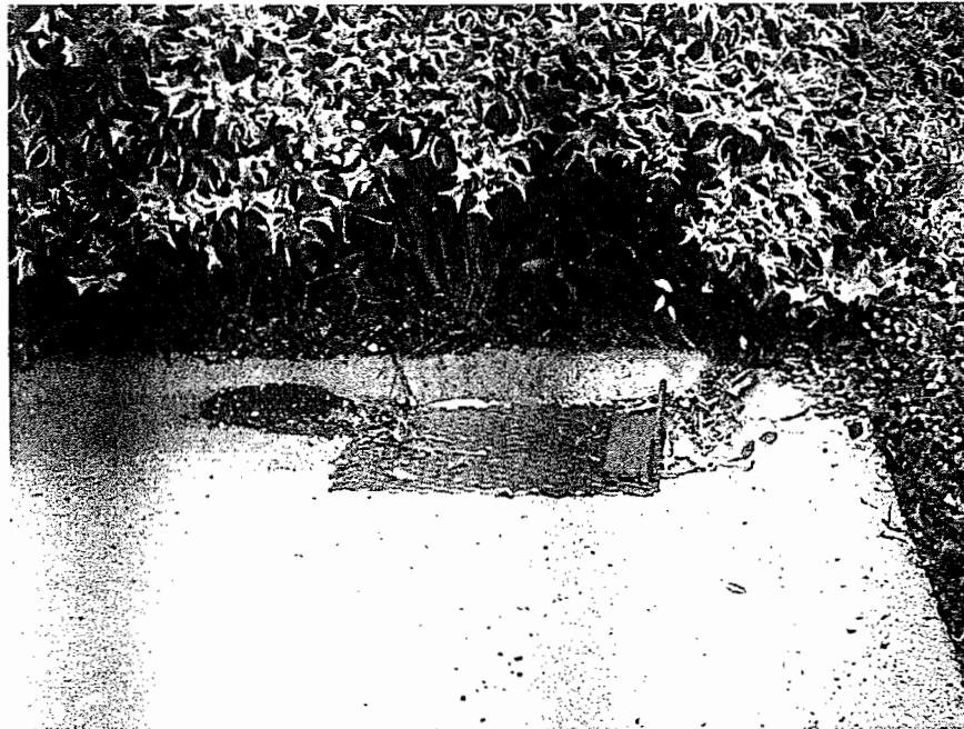
Photo 7 - Grate Cover over Flume C & D Outfall (12" PVC)
