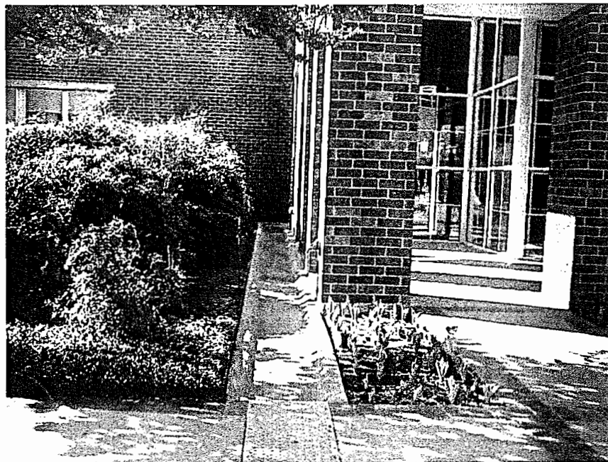
Photo 5 - Flume B, Entry Area
