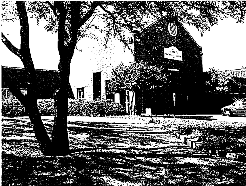
Photo 1 - Looking at Front Entry of Fire Station No. 1
