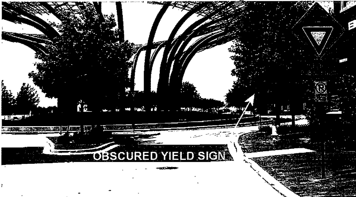
FIGURE 8: Westbound Obscured Yield Sign
