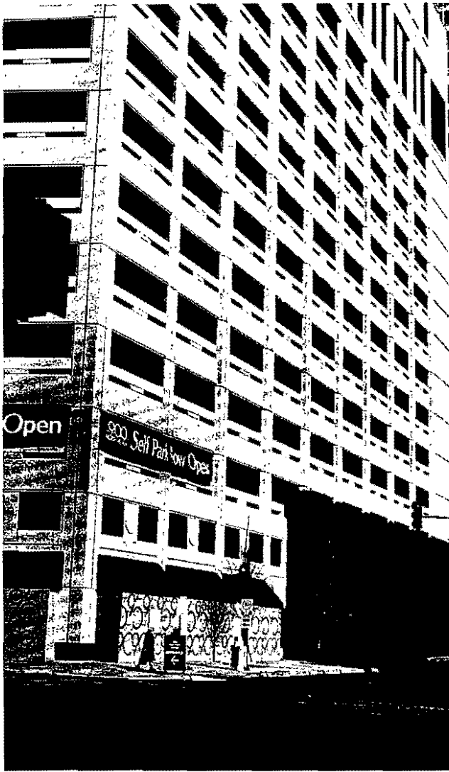
Parking garages are getting enormous. This garage, built to serve a new Bloomingdale's in Chicago, is 15 stories high and contains 1,450 parking spaces.
