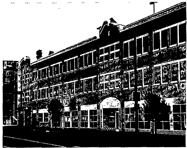
The design of the Schoolhouse garage in Pasadena, California, was the subject of 130 meetings of the city planning, design review, and cultural heritage commissions. (City of Pasadena, California, Public Works and Transportation Department)
