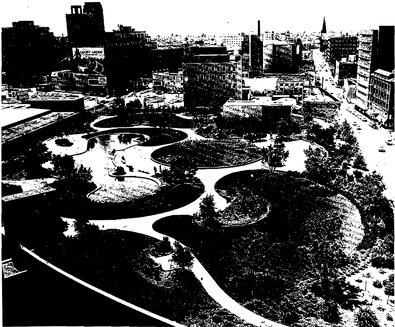
The nation's largest parking garage rooftop garden serves the Kaiser Center Building in Oakland, California. The garden atop this five-story, 1,500-space garage requires the care of three full-time gardeners and includes a reflecting pool built in the shape of nearby Lake Merritt. (Theodore Osmundson and Associates—Landscape Architects)
