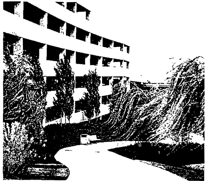
The columnar shape of these trees provides some relief from and contrast to the long horizontal lines of the parking garage.
