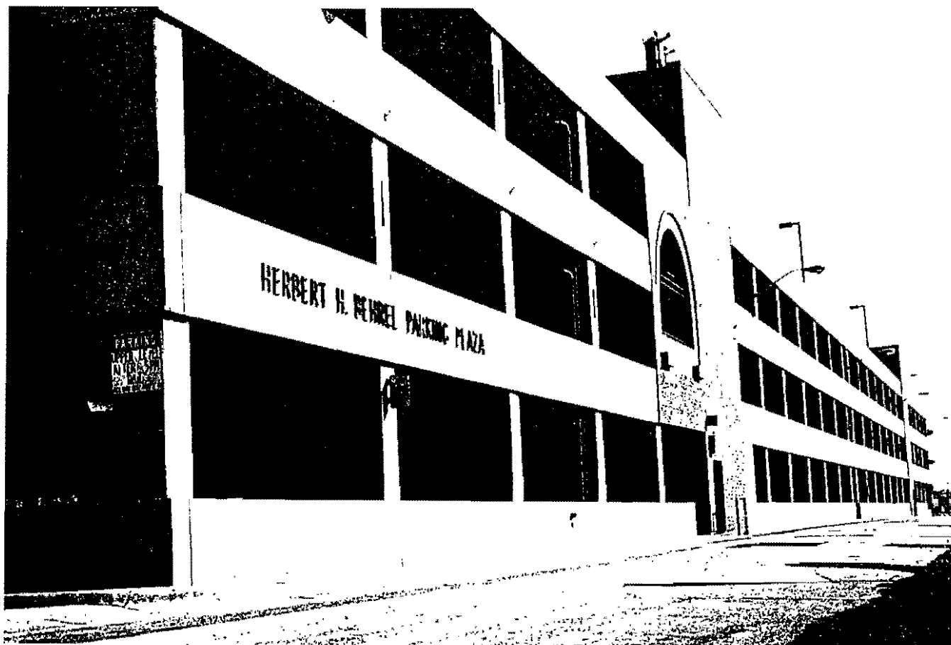
This garage in downtown Des Plaines, Illinois, has been called the Berlin Wall and a concrete casket. Local aldermen refer to it as "the zit."
