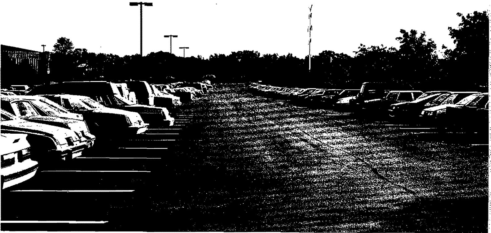
Some zoning codes require 90-degree parking and mandate excessively wide driving aisles. The result can be a waste of land and an excessive amount of asphalt. The driving aisles in this suburban office development are wide enough for landing a small plane.
