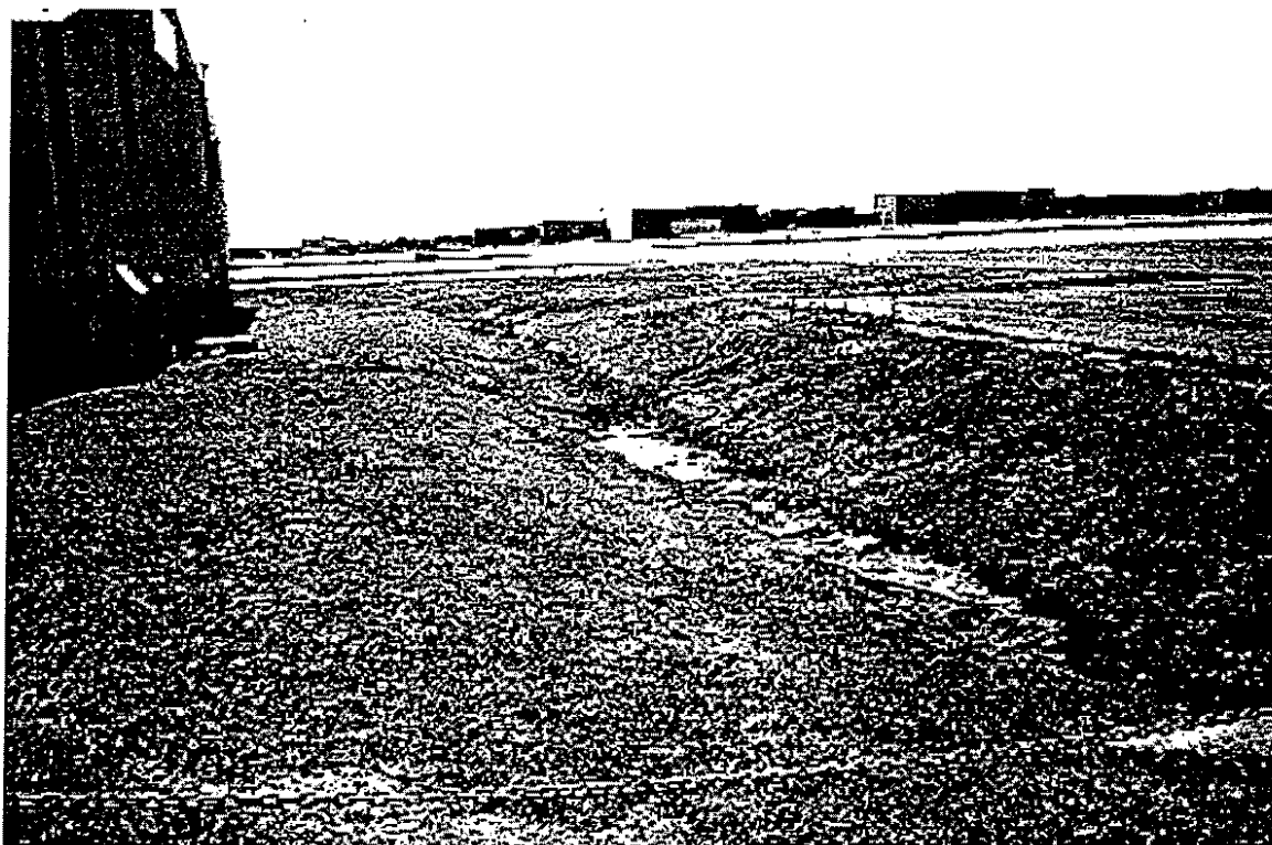
Photo 11: View of drainage ditch located west of remote dispenser. The ditch drains to a main drainage channel that flows to the southern end of the airport and enters the storm sewer system in the Lindberg Road right of way. View is to the west.
