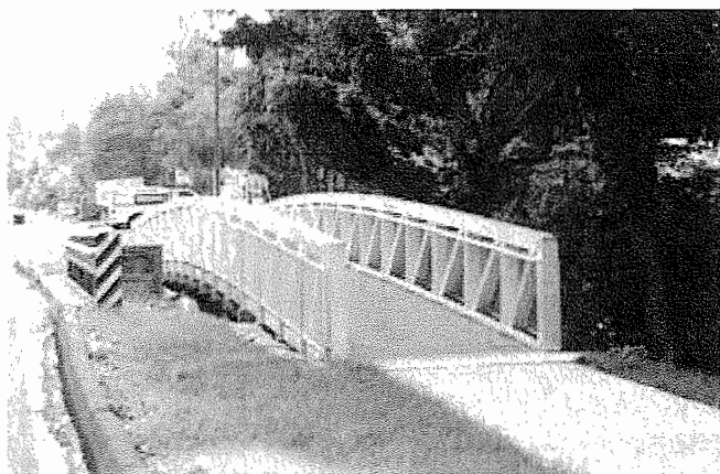
Pedestrian bridge next to highway. Volusia County, FL
