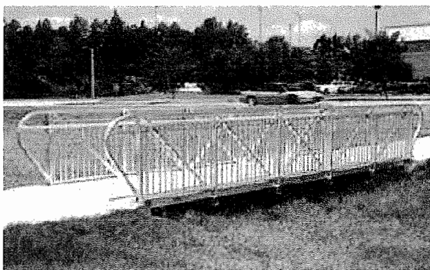
A 6' wide X 30' long bridge is used to span a retention basin.
