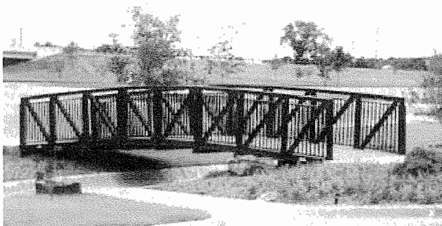
Dark Green painted bridge. N. Richland Hills, TX
