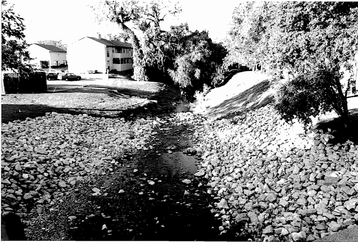
Downstream View Looking Southwest
