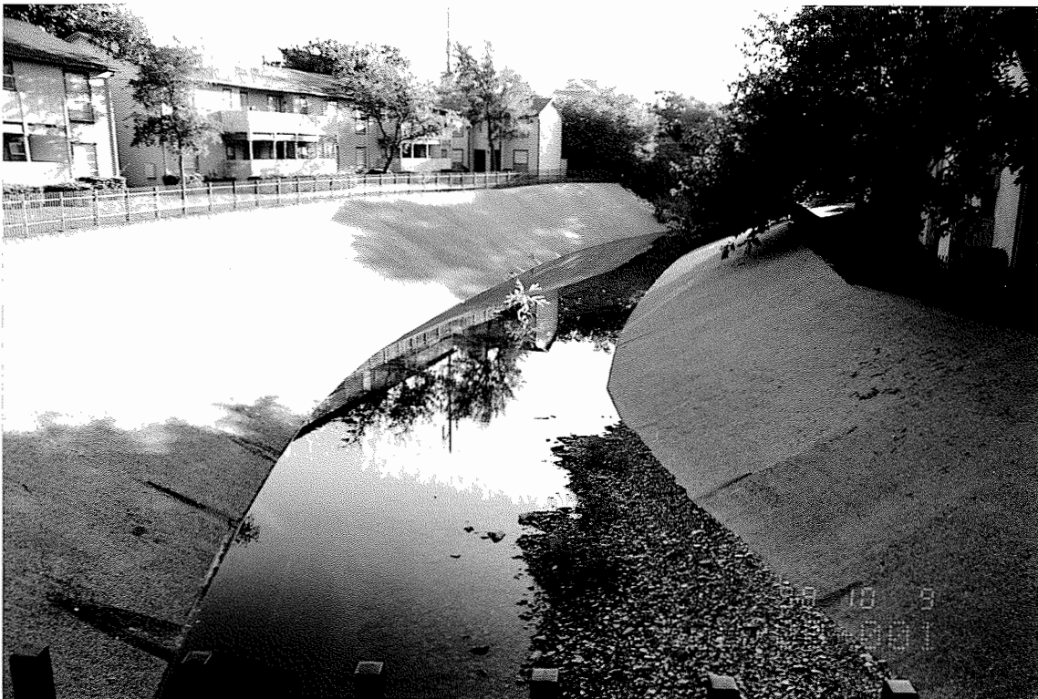
Upstream View Looking Northeast
