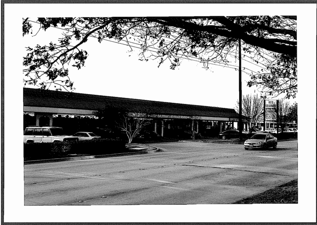
View of the subject from across Inwood Road, looking west.
