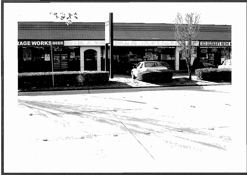
View of proposed DE-7 area from across Inwood Road.
