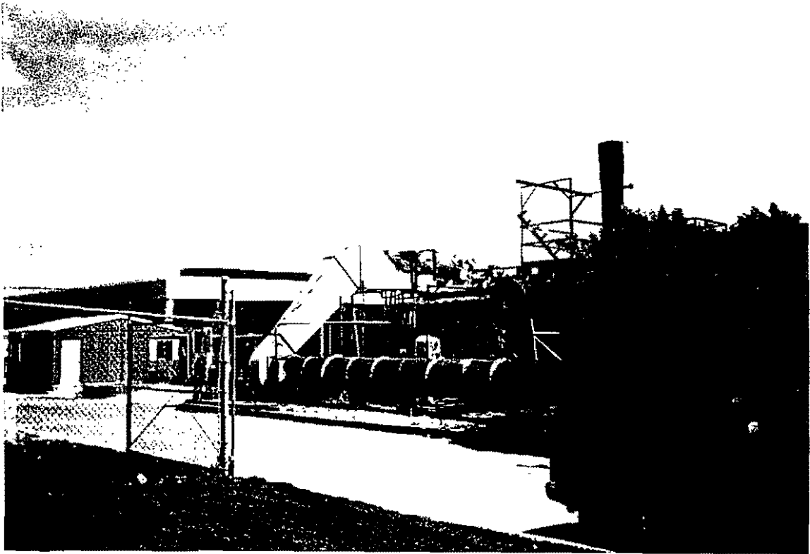
Photo 11 - View southeast of Forney Engineering diesel igniter testing facility for coal fired power plants.
