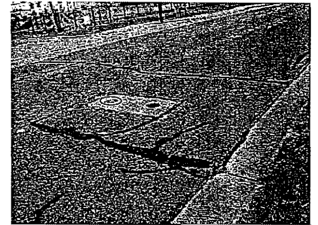
VALVE 20M2 ADDISON RD. (NB)
