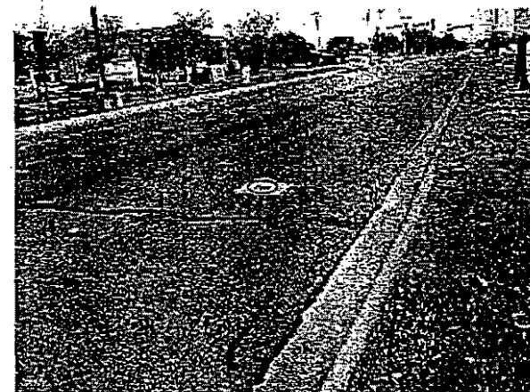
VALVE 20M5 ADDISON RD. (NB)
