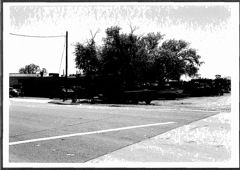
View from the railroad northeast of the subject looking SW; trucks on RR property.
