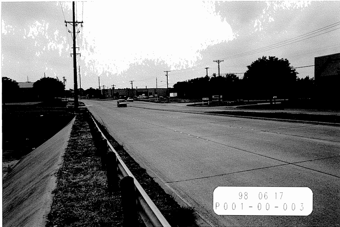
Roadway Over Bridge Looking South
