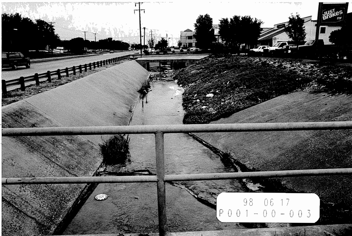
Upstream View Looking North
