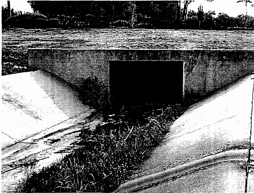
Photo 1 - Looking Upstream at Midway Culvert
