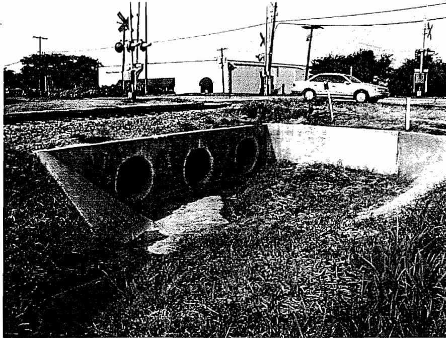
Photo 3 - Upstream side of Midway Road
