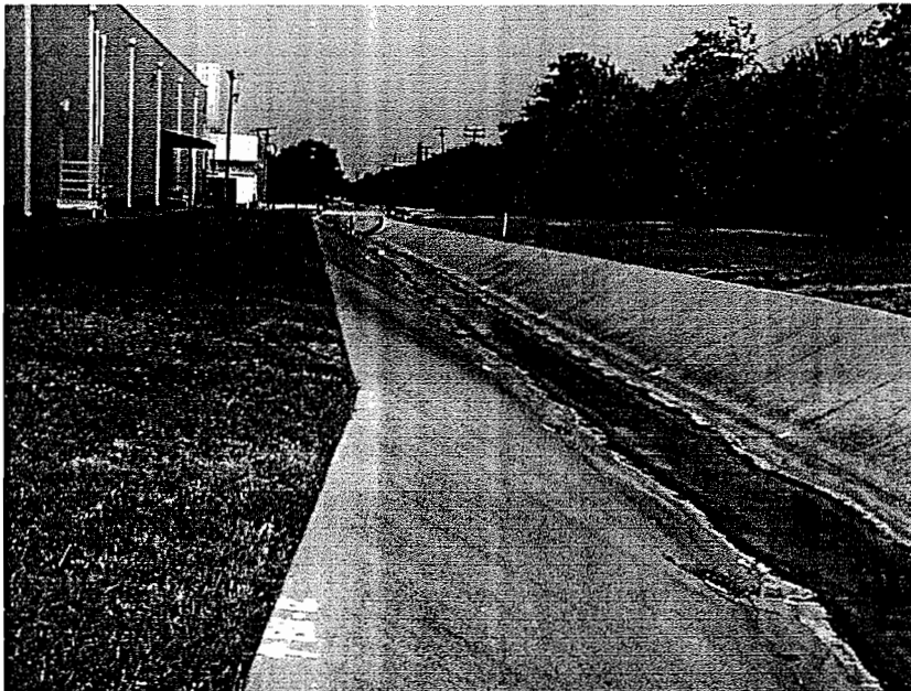
Photo 2 - Looking Downstream of Midway Culvert
