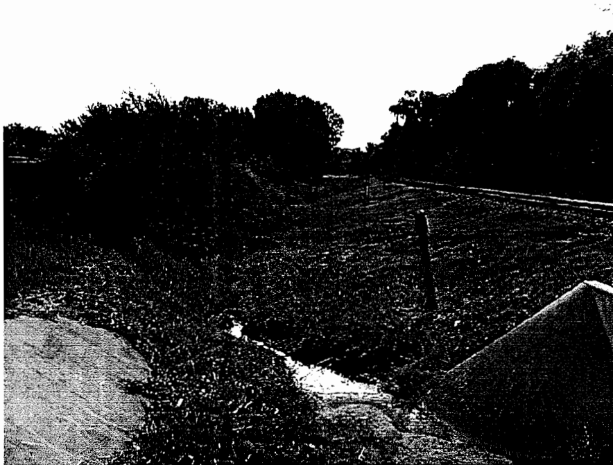
Photo 4 - Looking downstream from Midway Road
