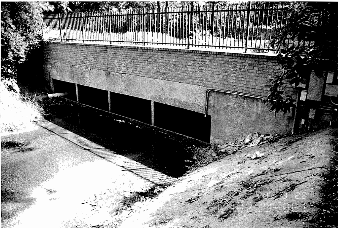
Elevation Looking Northeast
