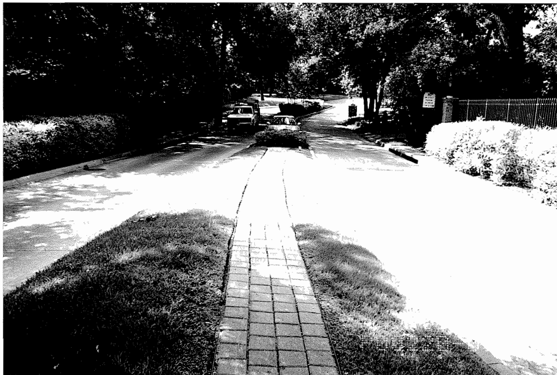
Roadway Over Bridge Looking South
