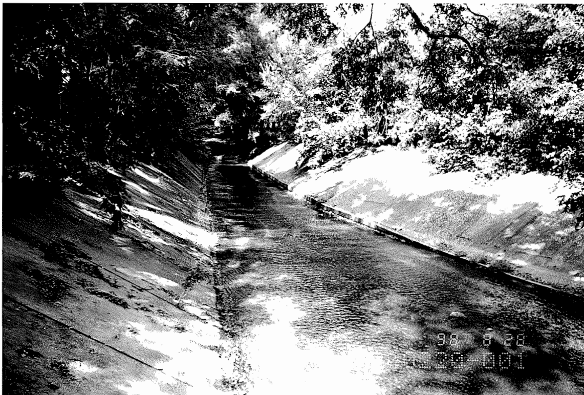
Upstream View Looking West
