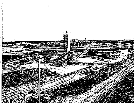
Biosolids —The biosolids staging facility has a capacity of 250 plus dry tons per day. Biosolids can be prepared at this location as either a class "A" or "B" material depending on its ultimate application.
