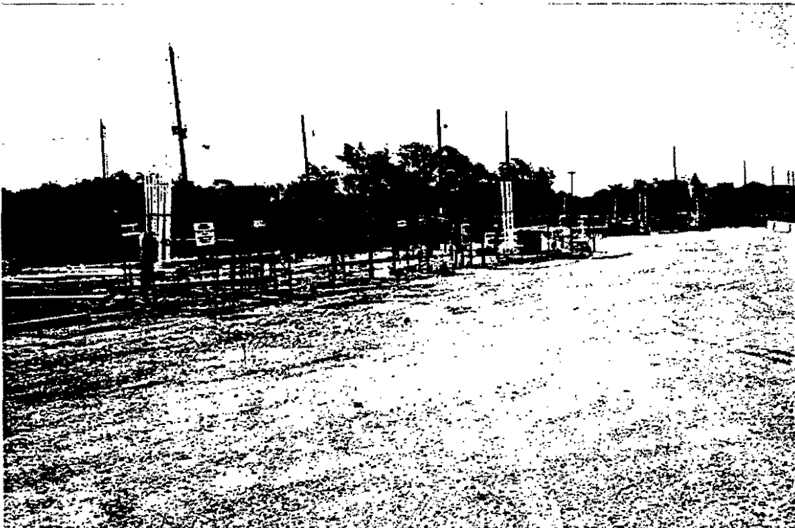
SUBJECT FUEL FARM IN FOREGROUND AND TWO ADJACENT FUEL FARMS IN BACKGROUND
