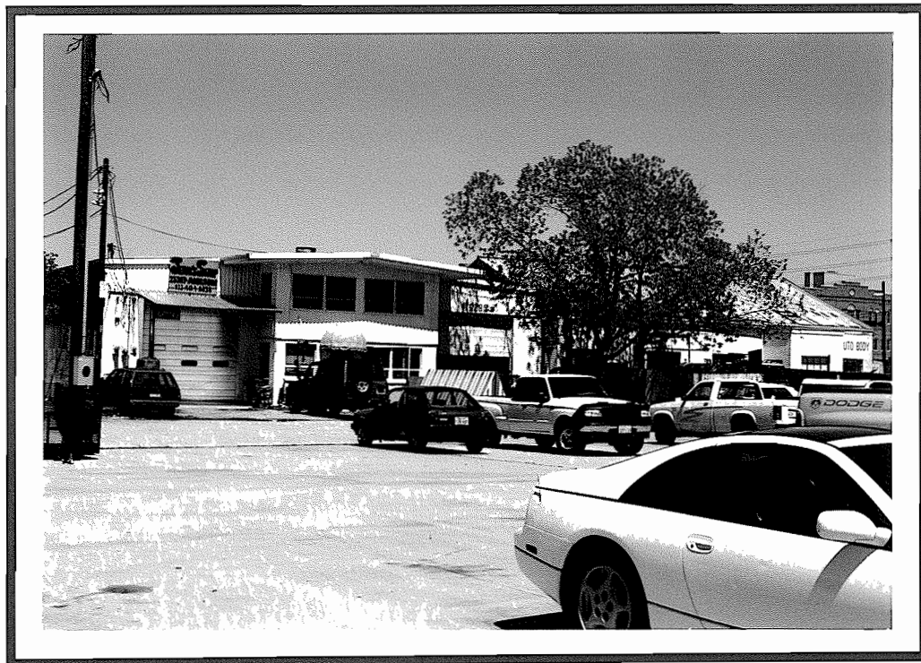
View of the south side of the partial 2 story building from site interior.
