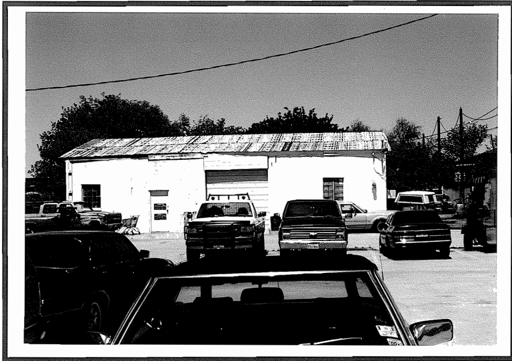
View of the smallest concrete block bld. near the northwest corner of the site.
