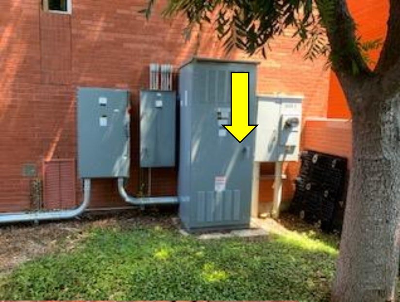
On the inside of the Chiller Unit.
