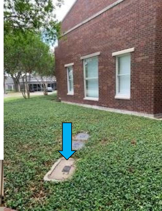
On the East side by Admin Offices
