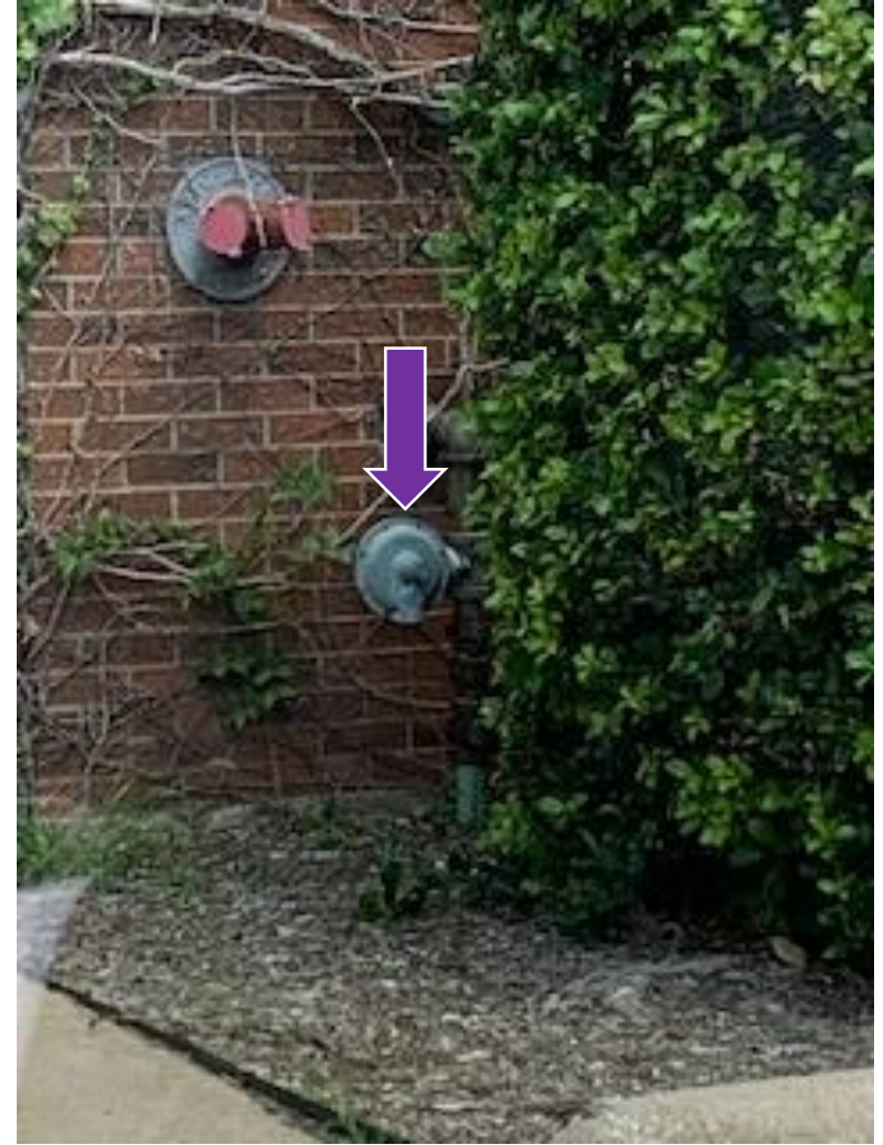
On Northwest corner of the building
