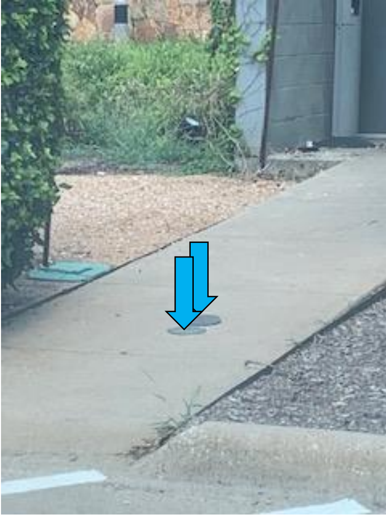
On Northwest corner of the building
