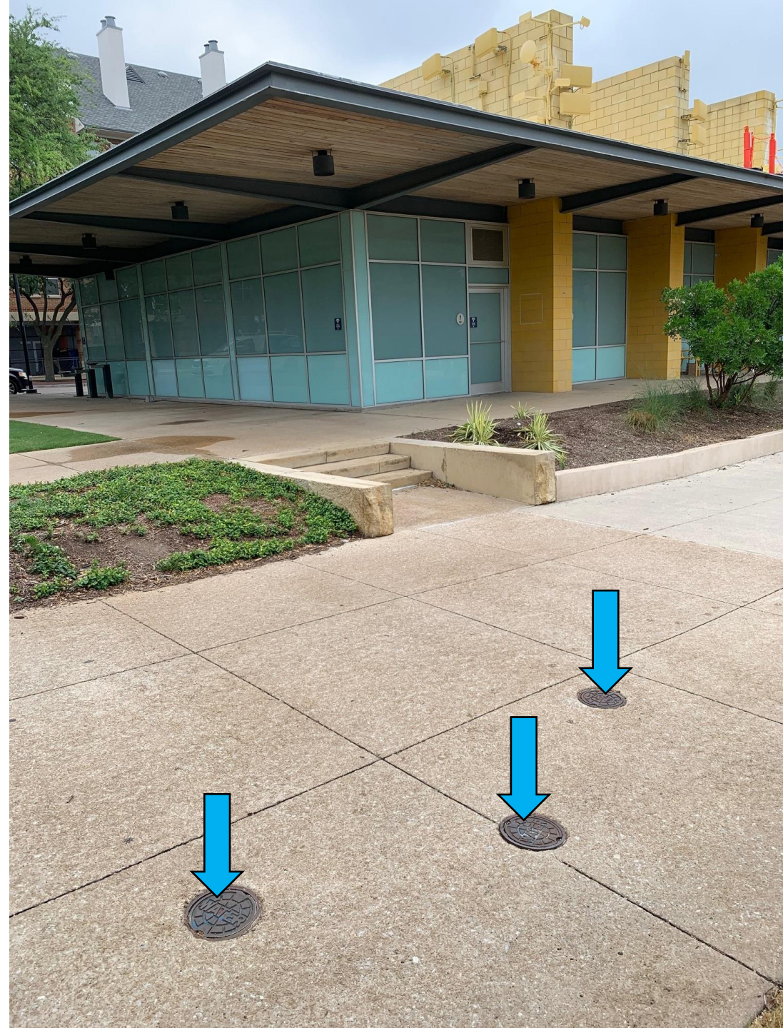
On the Southwest corner of the building
