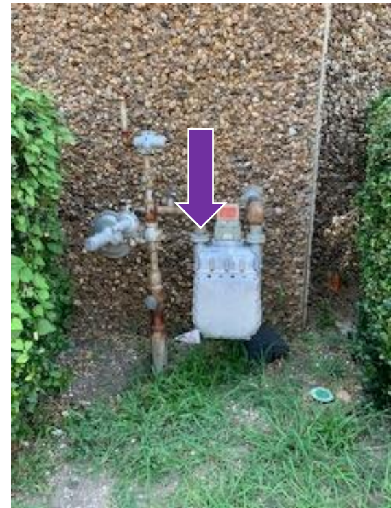
On the Northeast Corner of the building
