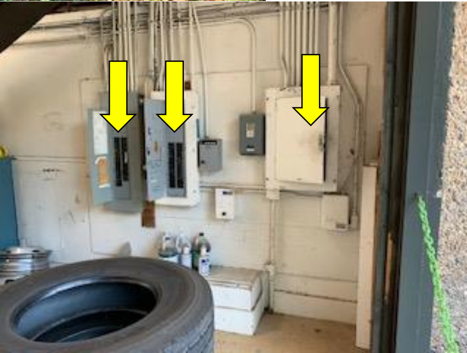
On the Northeast side of the Fleet Shop
