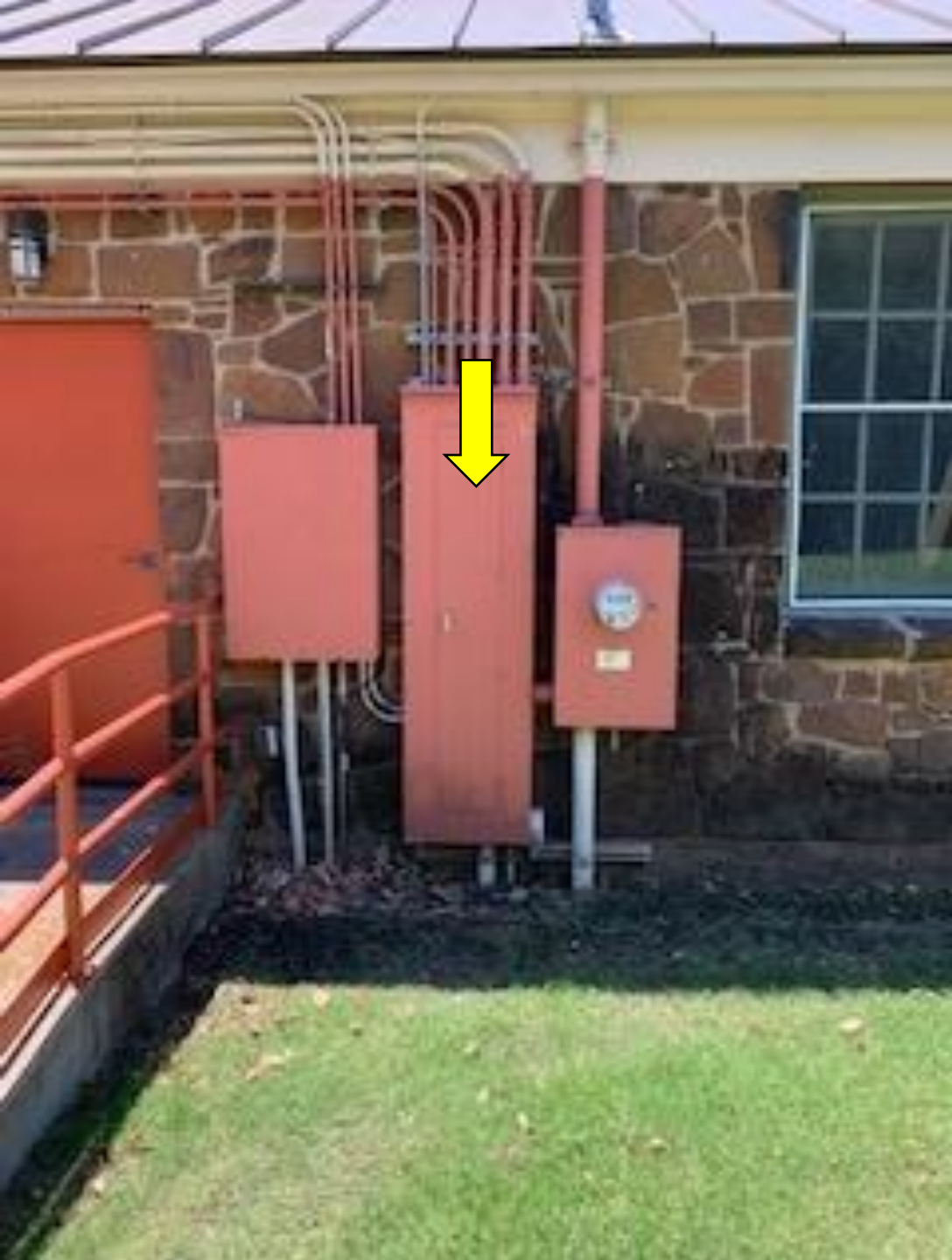
On North side of building
