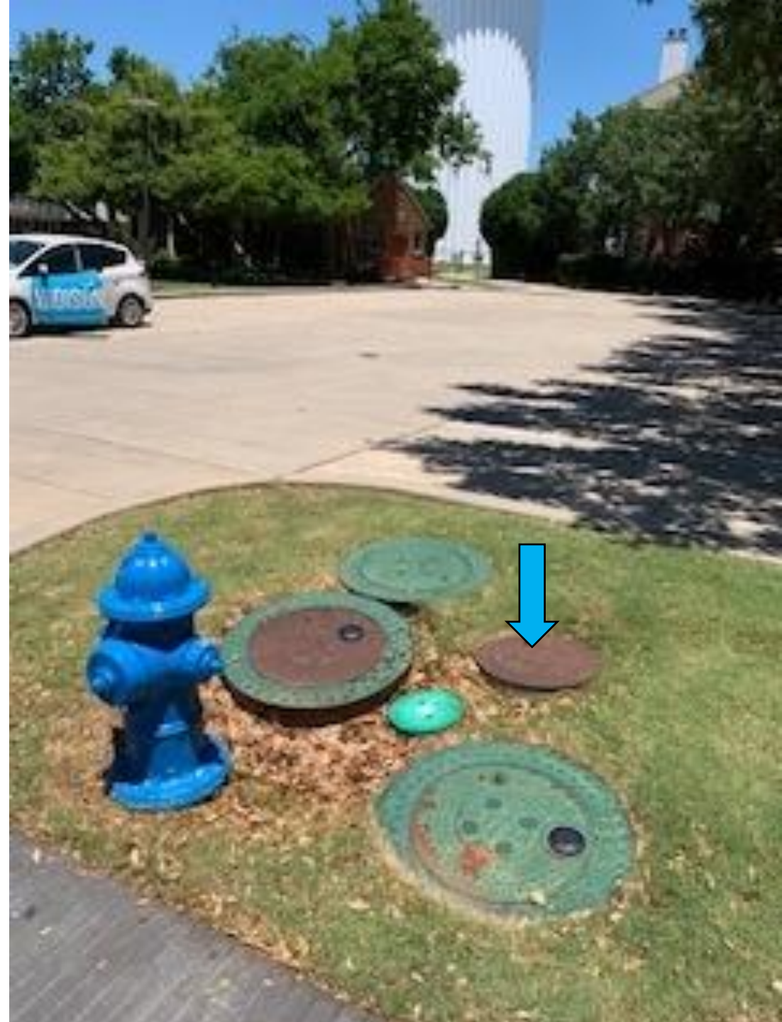
By hydrant next to Substation
