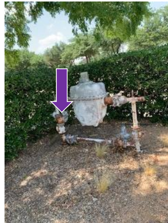
On Northwest corner of the building.
