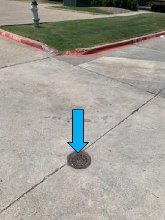
On Northwest Corner of the building. Main Feed.
