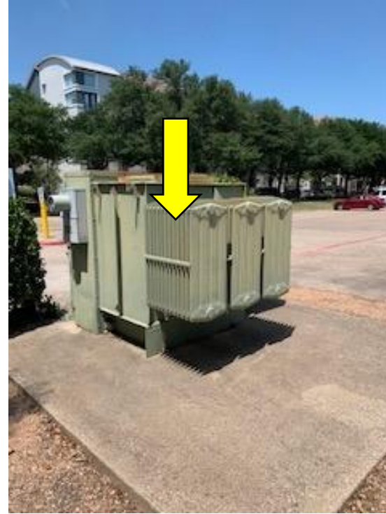
On Northwest corner of the building.
