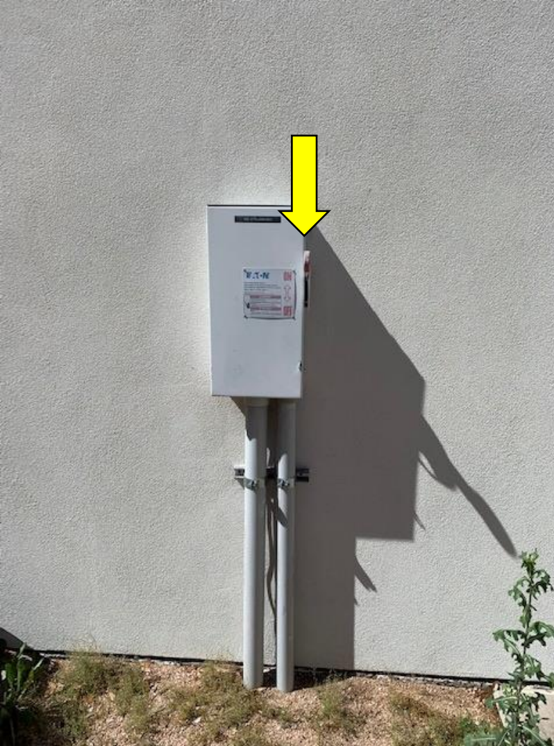
On North side of building in the gated area.
